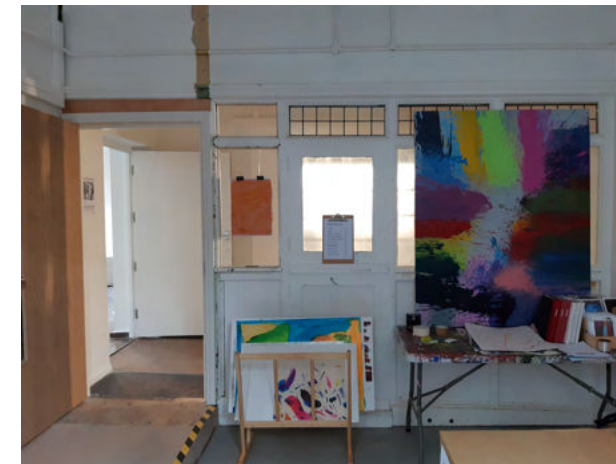
5. Circulation space: original timber and glazed screen and good levels of natural daylight
