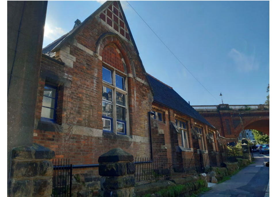
1. Existing view of Trinity Hall elevation from Braybrooke Terrace: the building has a strong street presence, framing the route to the Linton Road Bridge
