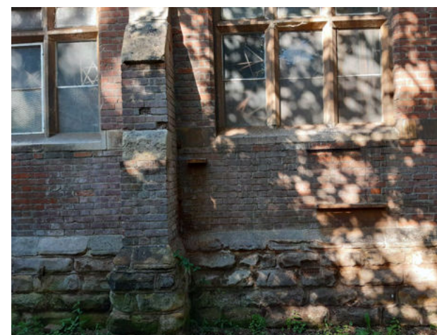
8. Existing structural piers and architectural features provide character along rear garden
