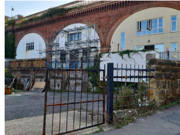
2. Existing main entrance from Braybrooke Terrace to yard space, overlooked by the Arches
