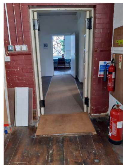
7. Changes in level and flooring is confusing
