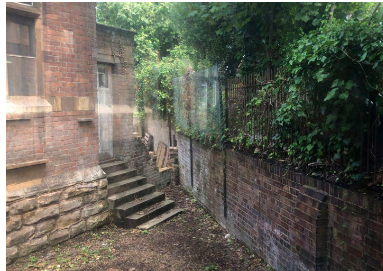
4. Change in level between Main Hall and rear garden compromises accessibility to space. Some evidence of subsidence
