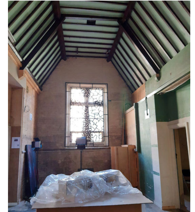
3. Small Hall looking North: double height space with vaulted soffit and exposed timber purlins
