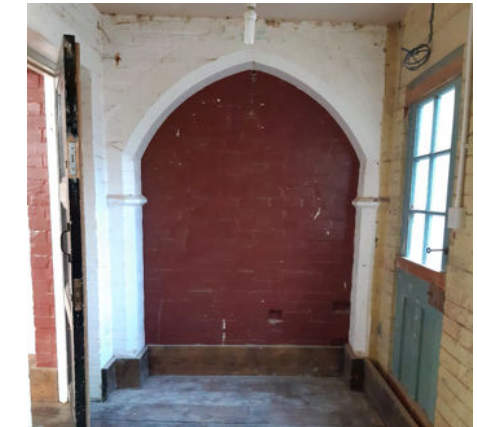
6. Original arched opening
